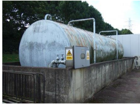
FIG.12. The bunding on this fuel tank not only prevents an uncontrolled spill but also acts a barrier between mobile plant and the tank
